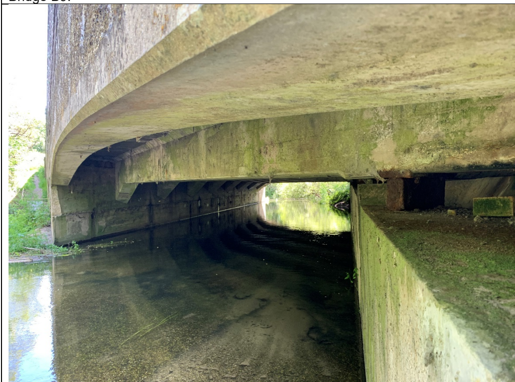
Photograph 8: View looking west on northern side of the river (Bridge B9)
