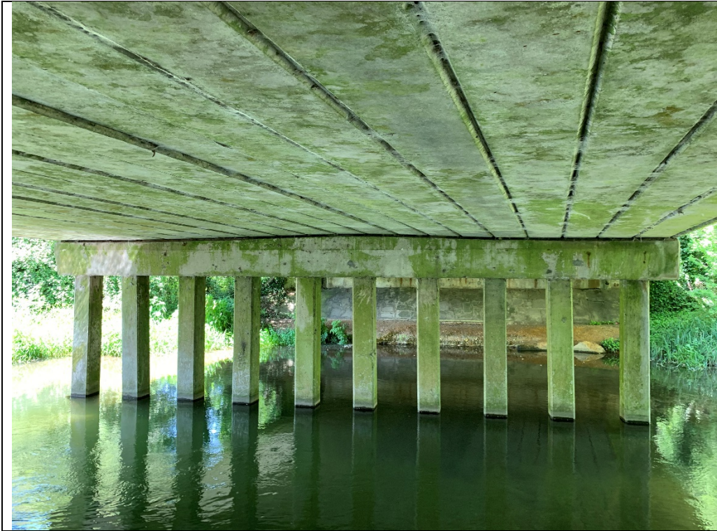
Photograph 1: Bridge B8 (concrete beam structure)
